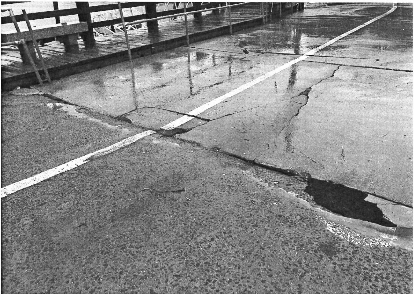
STONY CREEK WHARF- CONCRETE RAMP
