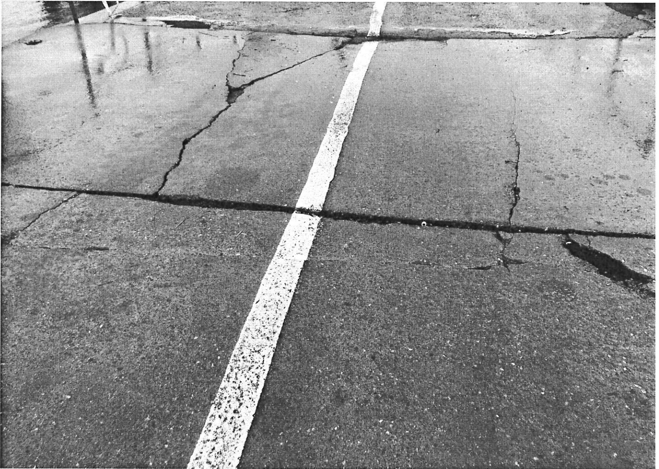
STONY CREEK WHARF- CONCRETE PIER
