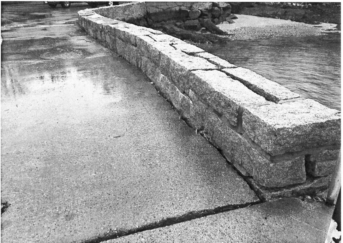
STONY CREEK WHARF- CONCRETE PIER
