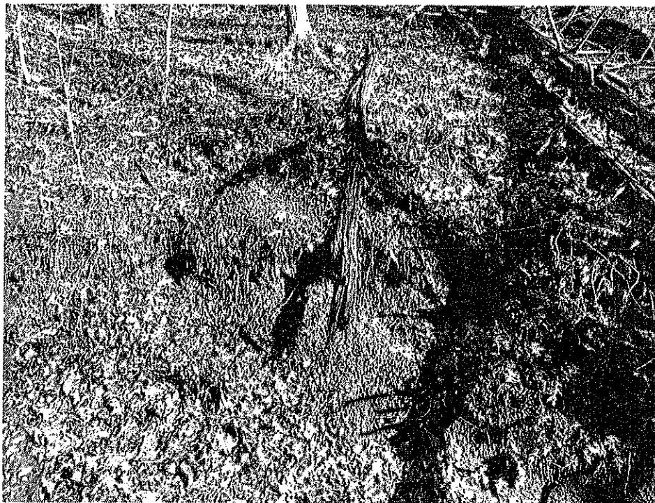
Photo 4: bank stabilization (dormant live stakes)
