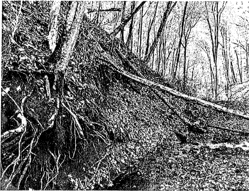
Photo 15: bank stabilization (dormant live stakes)
