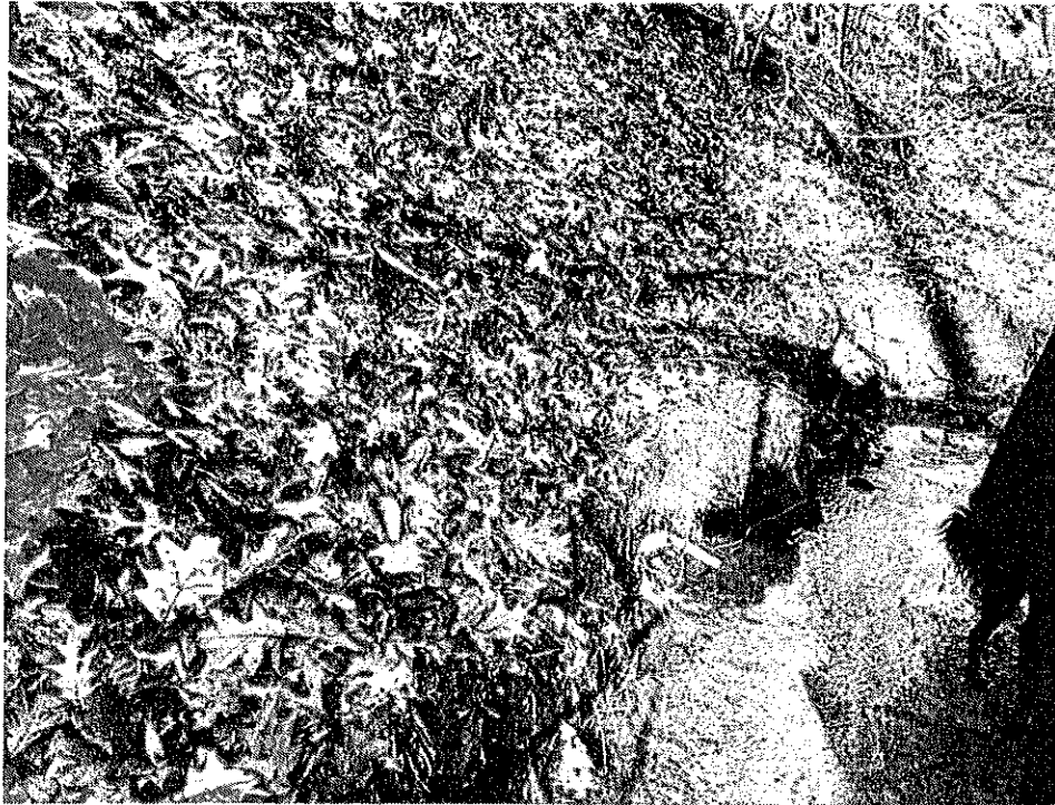
Photo 7: bank stabilization (dormant live stakes)
