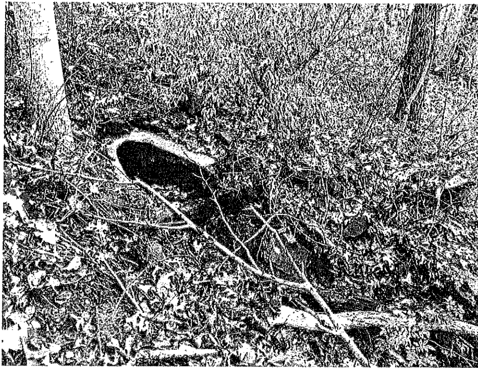
Photo 3: outlet protection (reconfigure with existing rip-rap)
