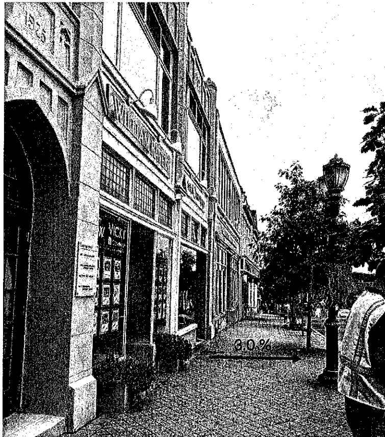
Figure 8. Example of non-ADA compliant sidewalk cross slopes.
