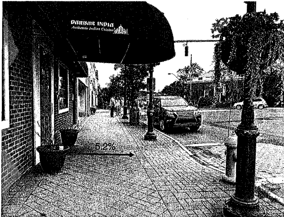
Figure 7. Example of non ADA-compliant sidewalk cross slopes.
