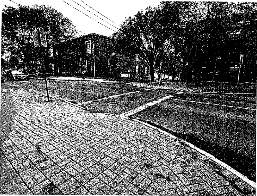
Figure 1. Representative photo of non-ADA compliant sidewalk ramps and crosswalks in poor condition.
