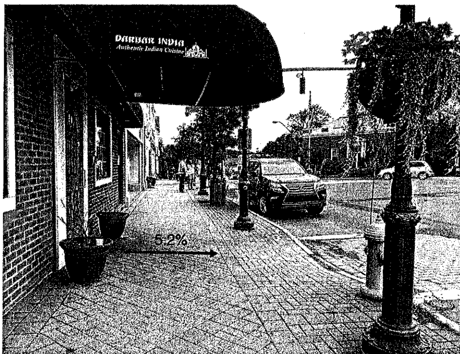
Figure 7. Example of non ADA-compliant sidewalk cross slopes.
