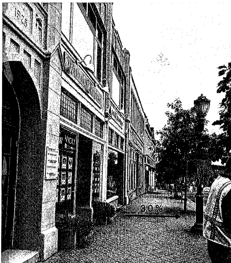
Figure 8. Example of non-ADA compliant sidewalk cross slopes.
