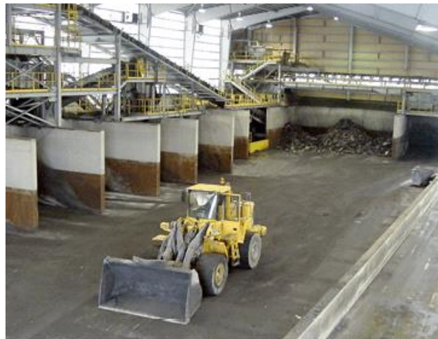
Ash processing and transfer station designed and built by RRT in Florida
