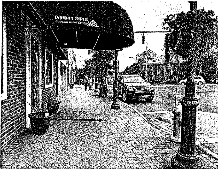
Figure 7. Example of non ADA-compliant sidewalk cross slopes.
