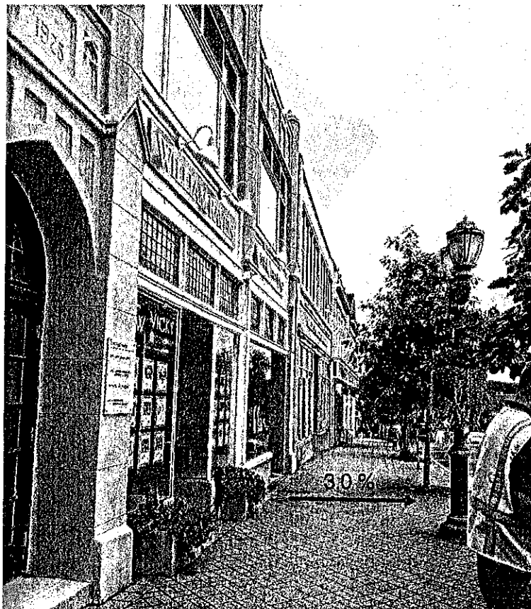
Figure 8. Example of non-ADA compliant sidewalk cross slopes.
