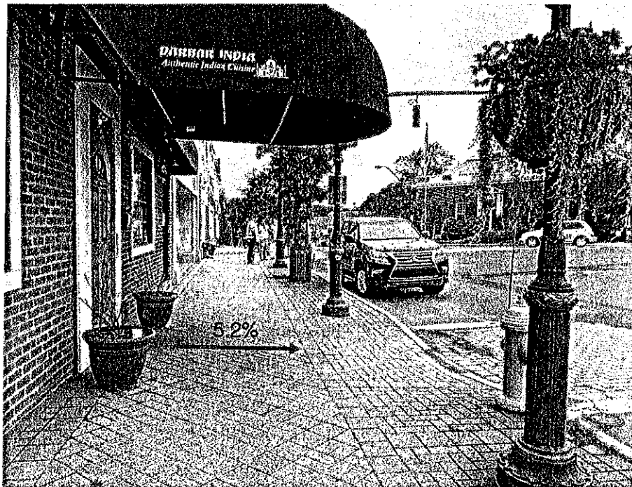
Figure 7. Example of non ADA-compliant sidewalk cross slopes.
