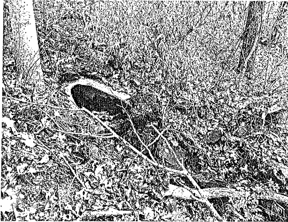
Photo 3: outlet protection (reconfigure with existing rip-rap)
