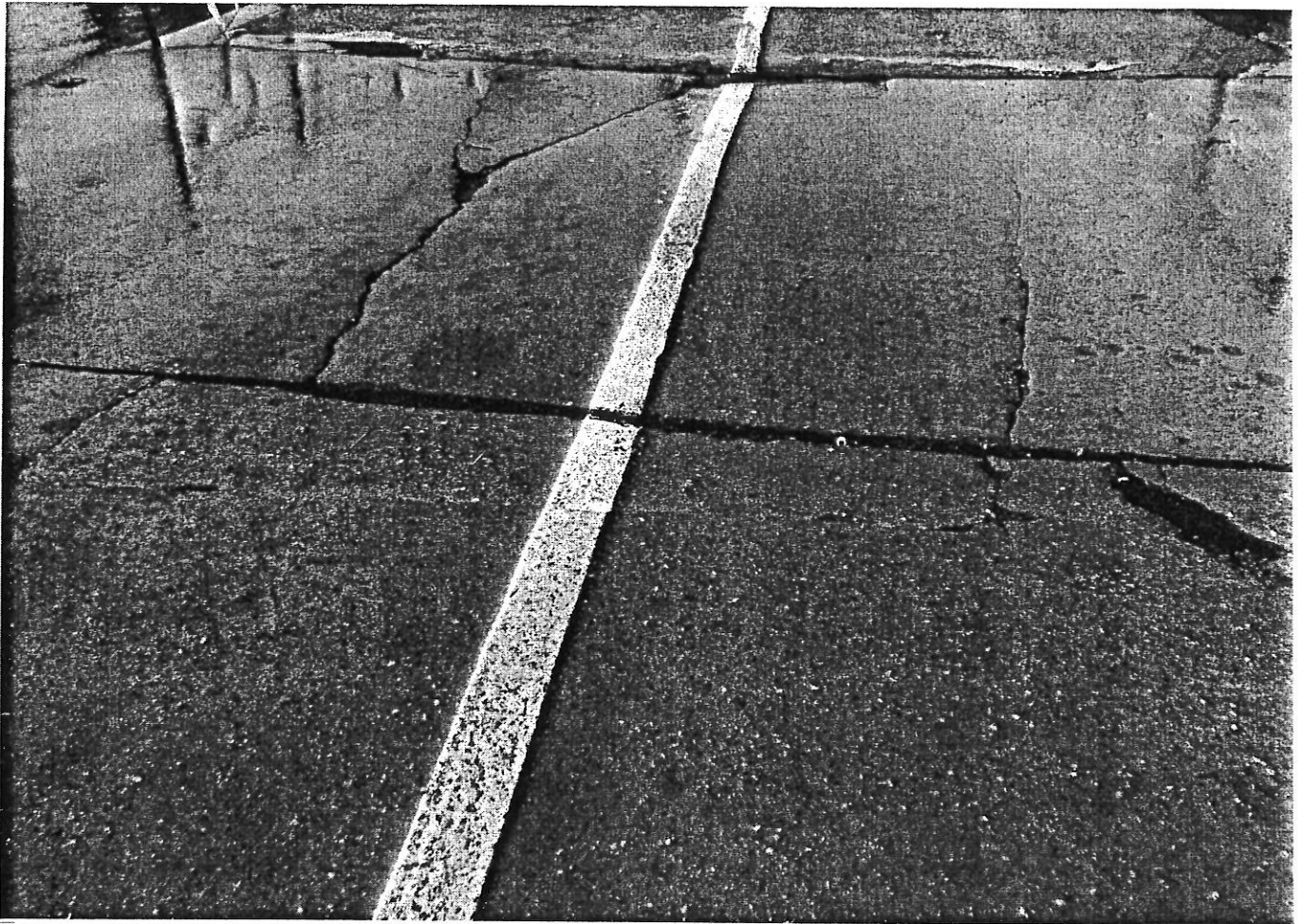
STONY CREEK WHARF- CONCRETE PIER
