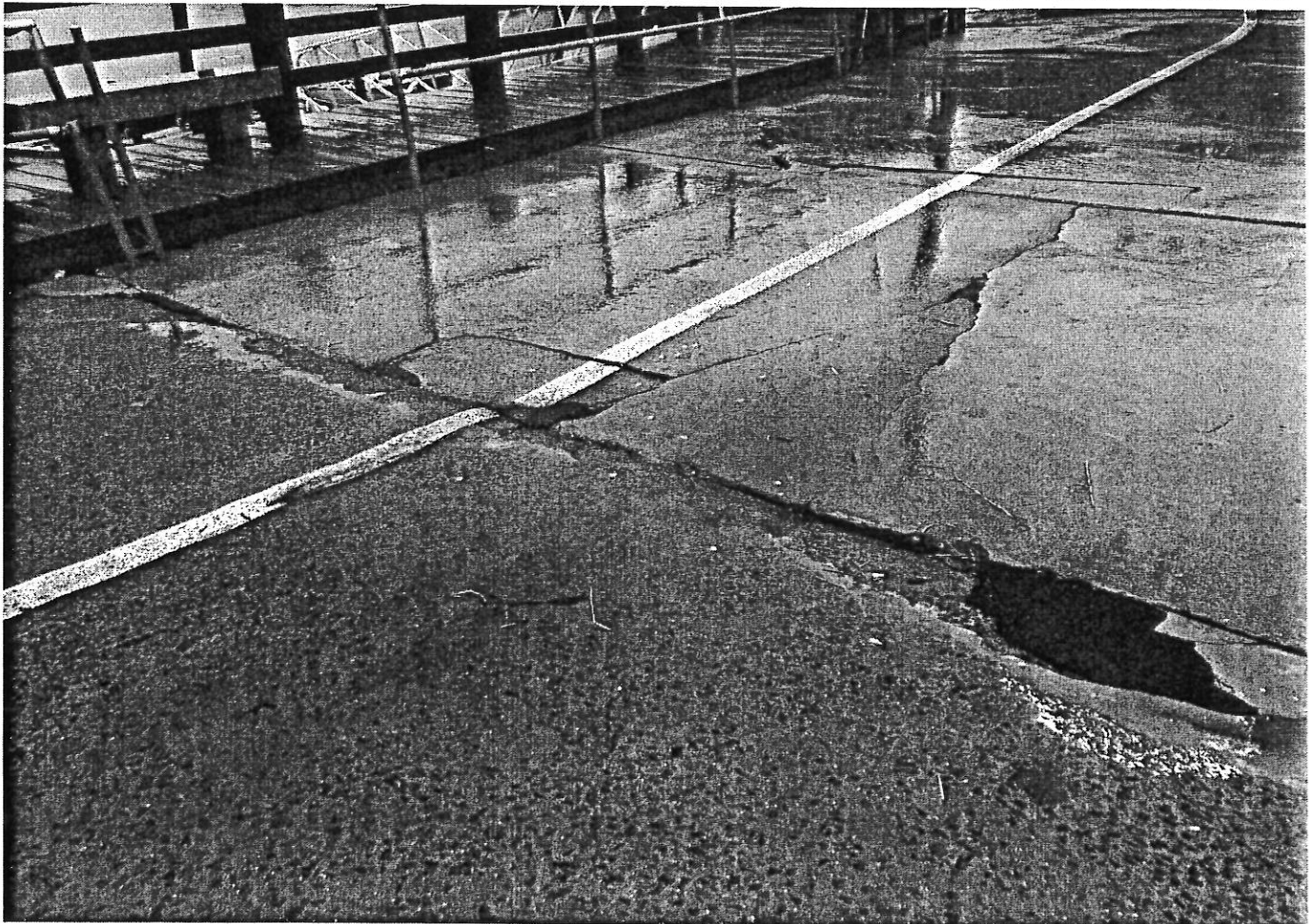
STONY CREEK WHARF- CONCRETE RAMP
