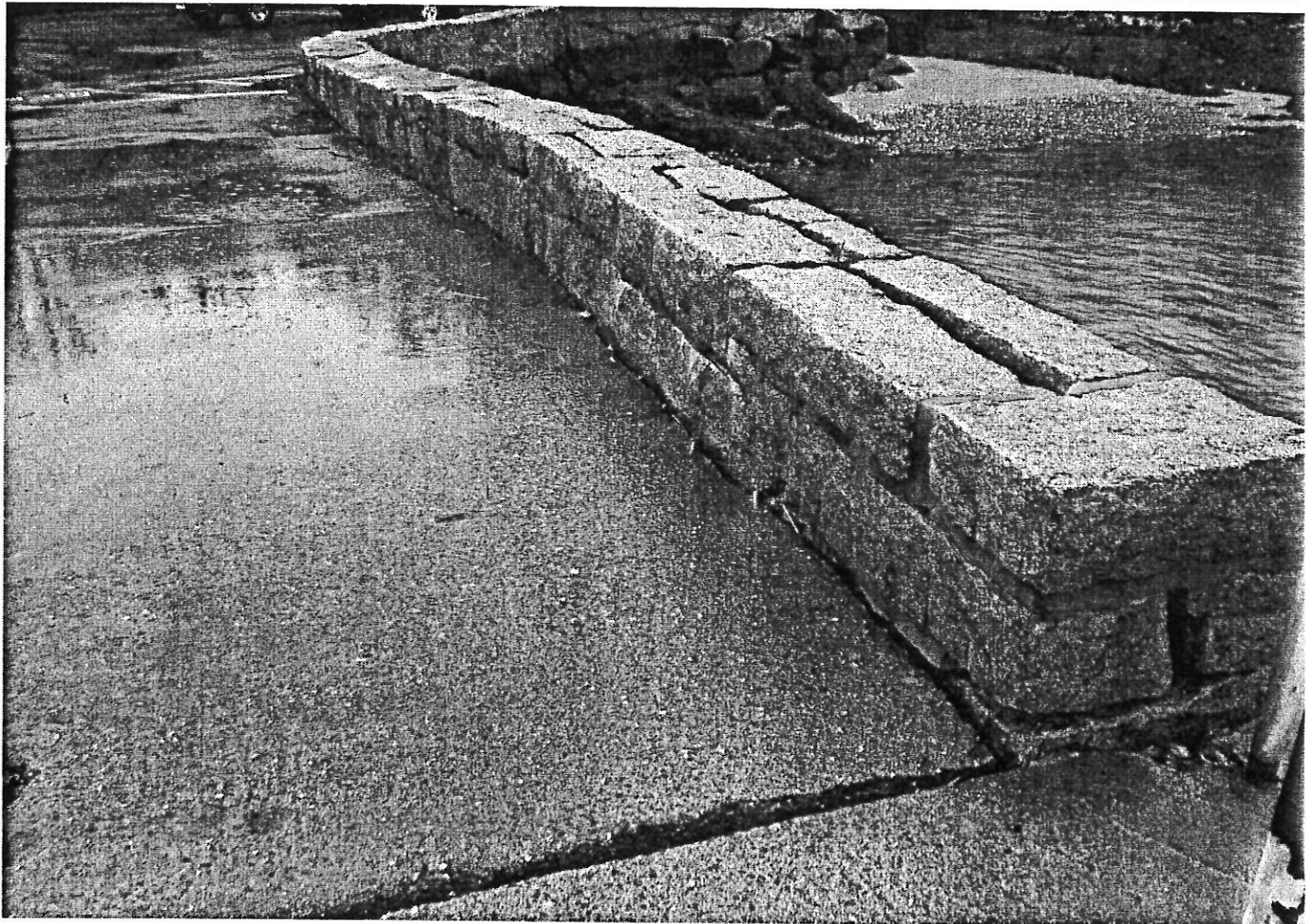
STONY CREEK WHARF- CONCRETE PIER
