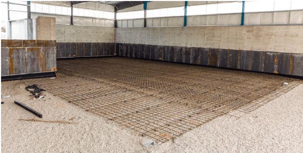
Organics processing and transfer facility designed and built by RRT in Ontario, Canada
