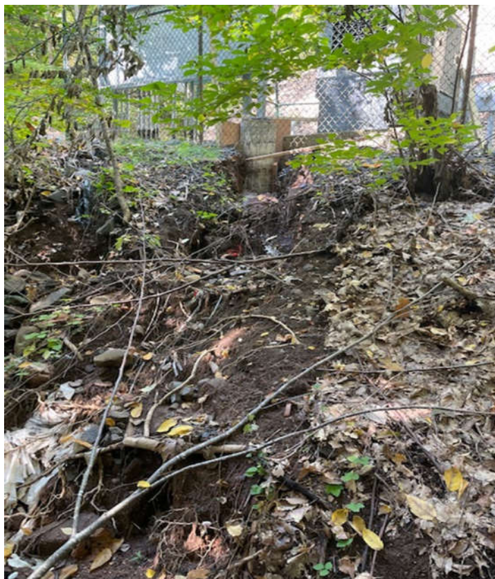
Unchecked Erosion Behind Squire Hill Pump Station
