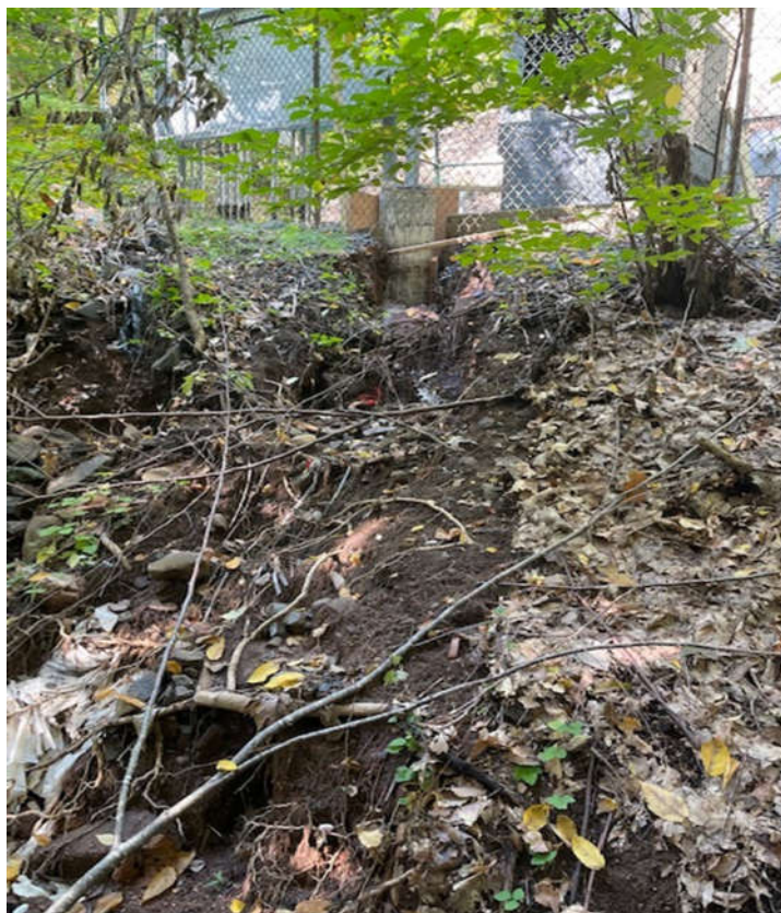
Unchecked Erosion Behind Squire Hill Pump Station
