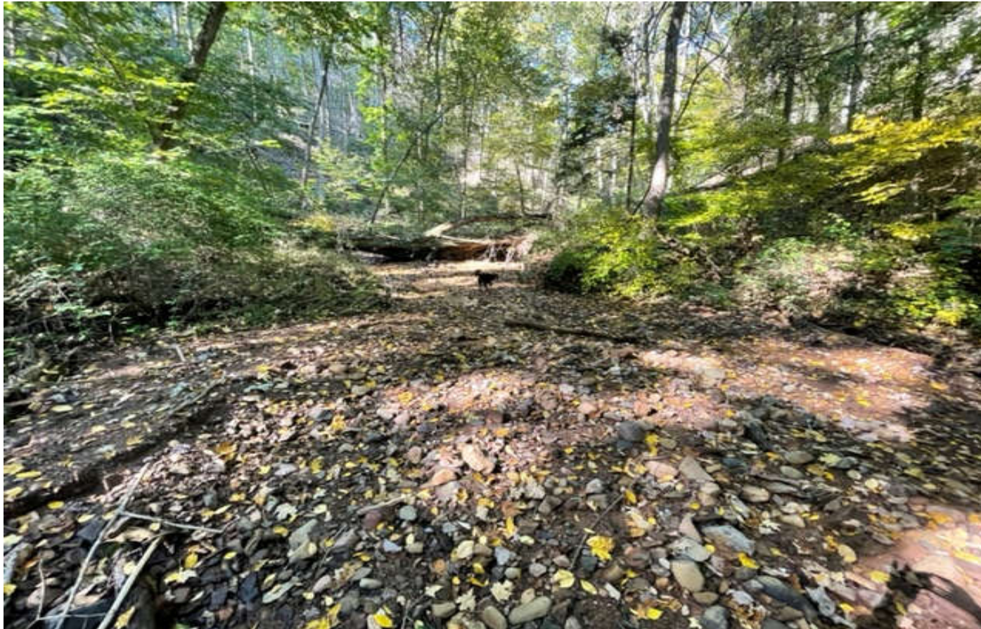
Major Erosion (Bank to Bank)
