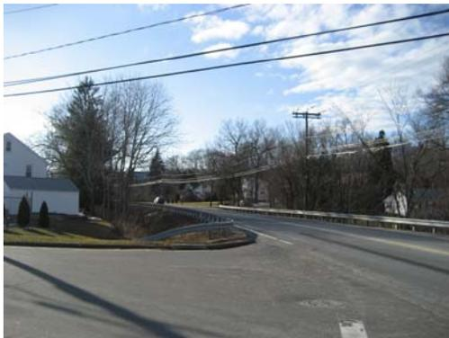
Chestnut Street – Visibility from the northbound approach of Chestnut Street at North Main Street is poor due to grade issues, a curve in North Main Street and an awkward horizontal alignment at the intersection. High prevailing travel speeds in this area have raised concerns over accident potential. Re-aligning the intersection would not be cost effective due to engineering constraints and right-of-way limits. Volumes at this intersection are not expected to meet signal
