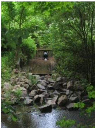
Pine Gutter Erosion Control Project
