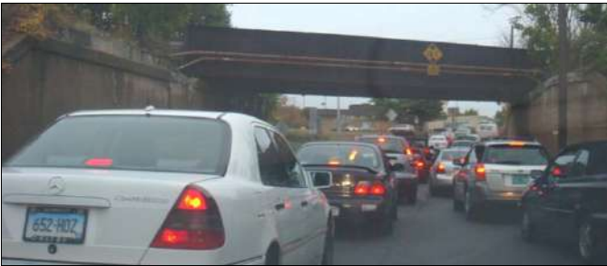
Route 1 railroad overpass
