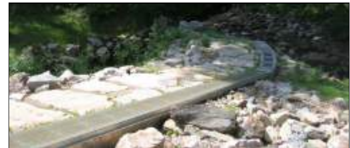
Supply Pond Fishway
