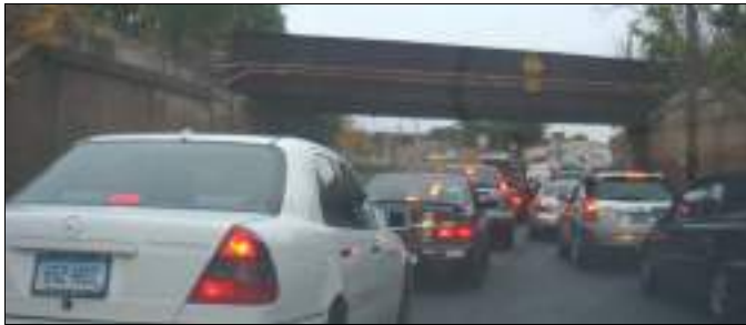
Route 1 railroad overpass
