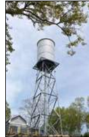
Stealth Installation In Branford
