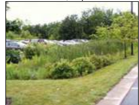
Water Quality Basin
