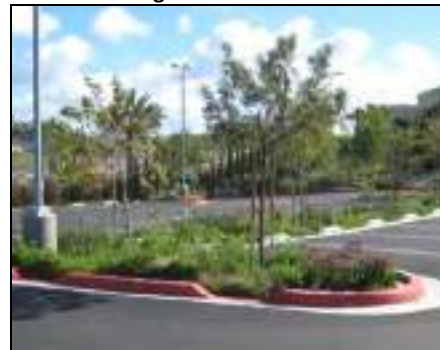
Parking Lot Infiltration Basin
