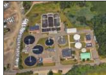
WPCA Treatment Facility
