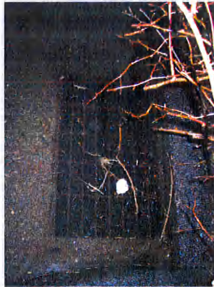
Figure 2.4. Overflowing storm drain during storm (April 2004).
