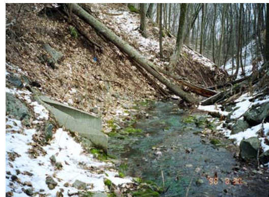
Figure 25. Discharge location of WS-60. 30" RCP with concrete and riprap bed armor.
