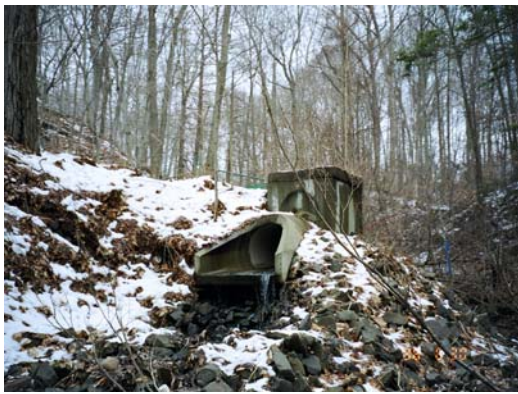
Figure 22. Discharge location of WS-30. Pipe is perched above grade.
