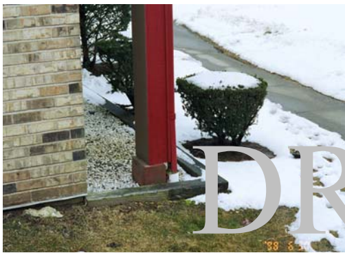
Figure 27. Downspouts at Squire Hill Apartment Complex are connected directly to the storm drainage system. This condition was observed at many residential properties in the watershed
