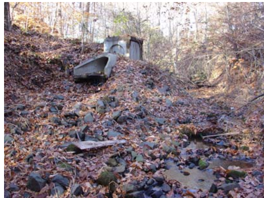
Figure 10. Perched storm drainage discharge in Reach 4.
