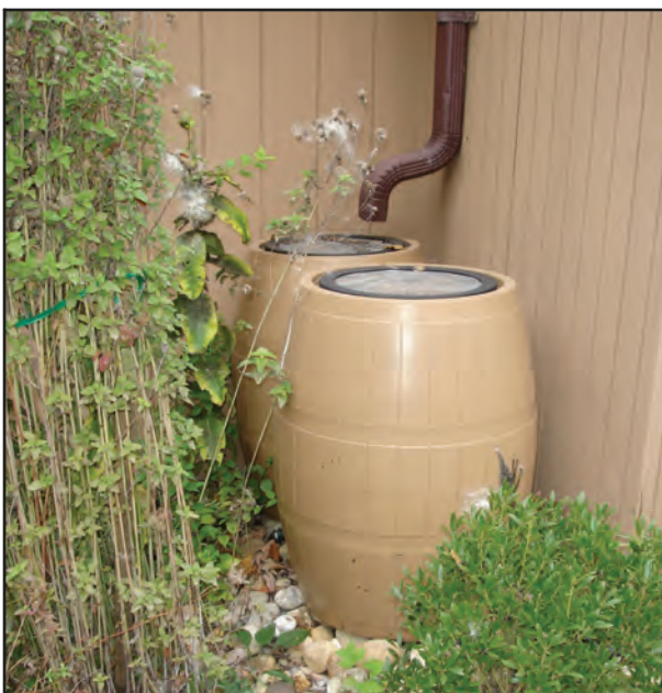
Figure 37. Connected rain barrels at Arlington Echo.
