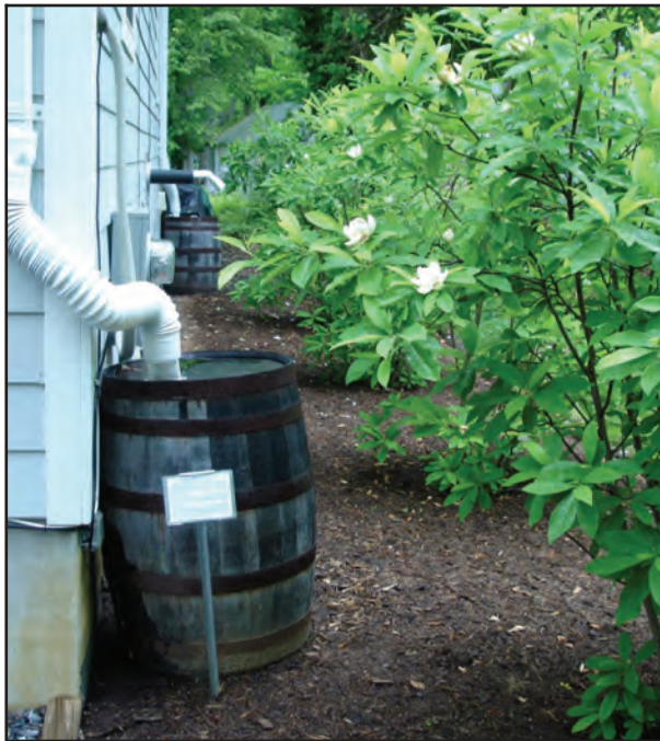
Figure 36. Highland Beach Town Hall rain barrels.
