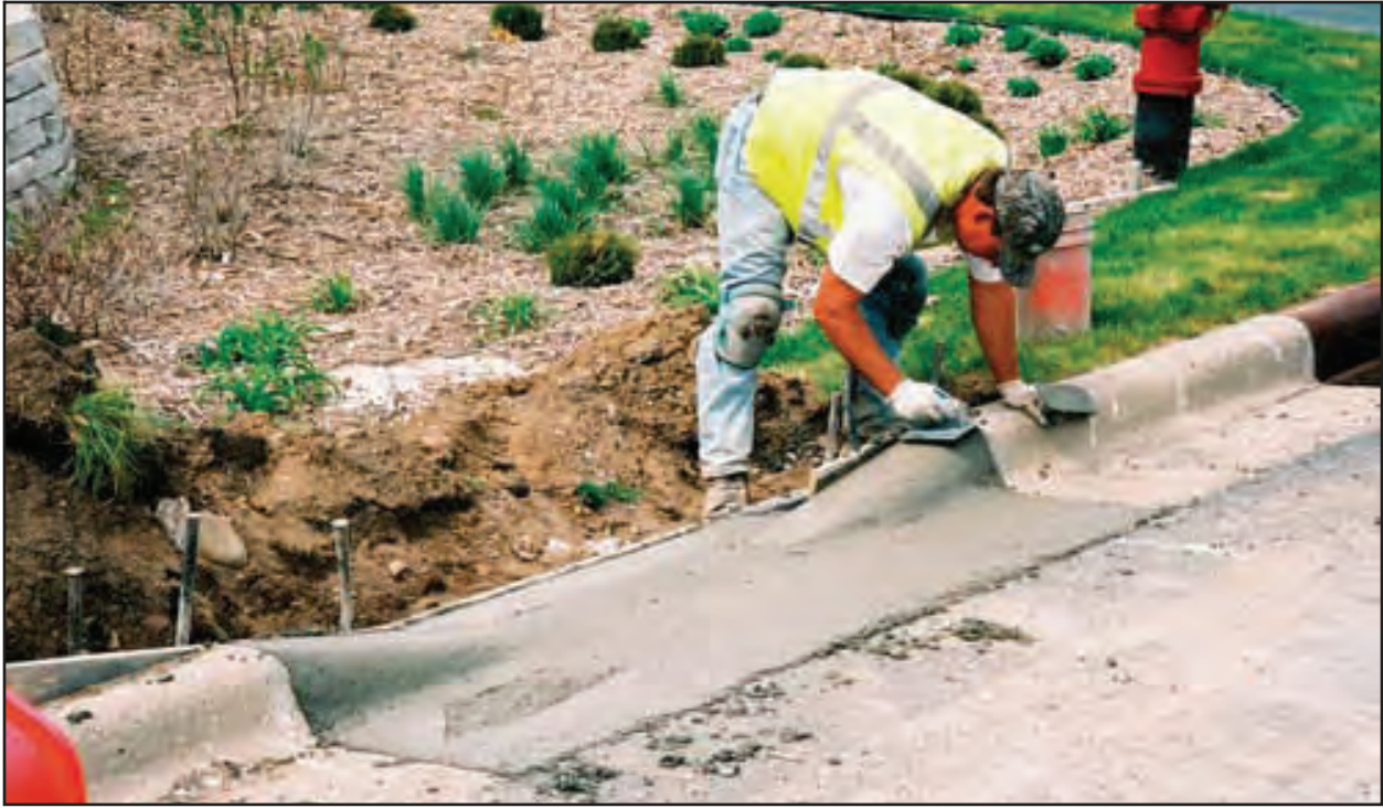
Figure 21. Creating a curb cut allows stormwater runoff from streets to enter rain gardens.
