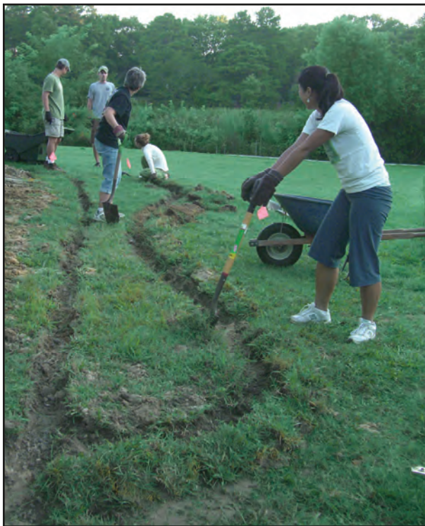
Figure 24. To construct the rain garden at the Ward Museum of Wildfowl Art in Salisbury, Maryland, the Lower Eastern Shore Tributary Strategy Team reused the garden area's sod to build a vegetated berm along the downslope side of the garden.
