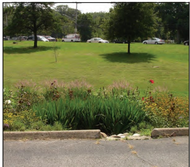
Figure 22. A curb cut allows runoff to flow into a rain garden at Heritage Baptist Church in Annapolis, MD.
