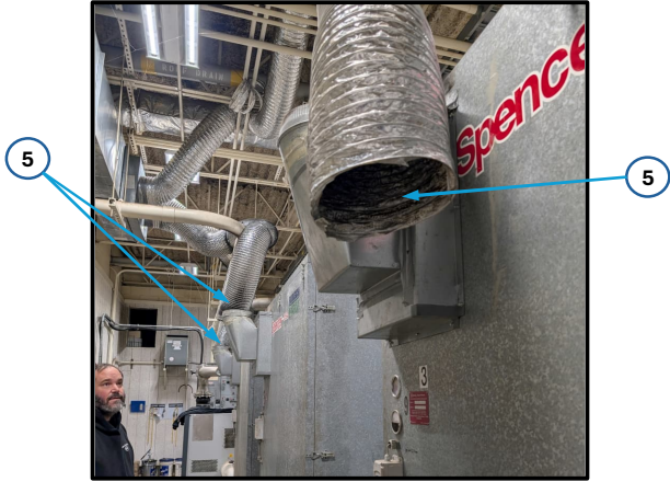
AERATION BLOWER EXHAUST DUCTWORK SCALE: NTS
