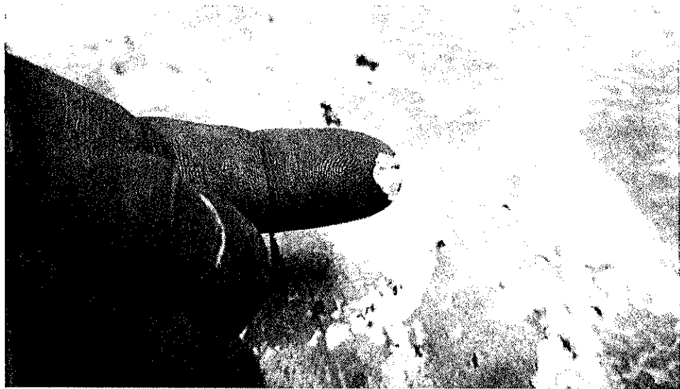
Photo 16 - Adhesive bonding vinyl tiles to blue coating was wet, deteriorated, and paste consistency.
