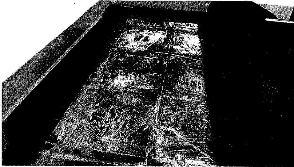
Photo 10 - View of resilient rubber floor rolled back to expose VCT.
