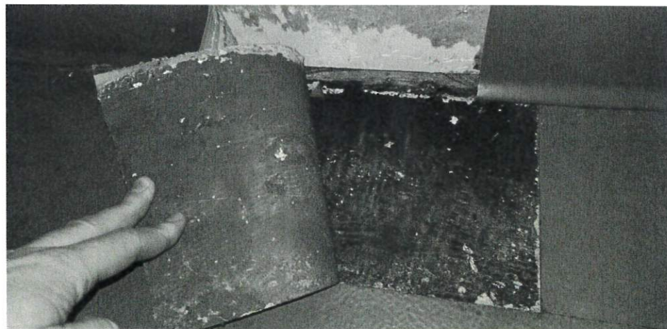
Photo 2 - View of solid vinyl tile, lifted. Note: blue membrane underneath.
