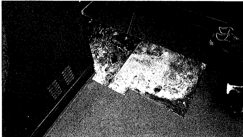
Photo 13 - Vinyl tiles removed in supervisor's locker room. Note: blue coating on slab.
