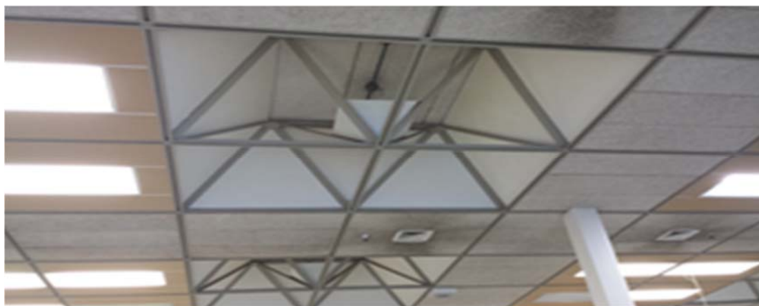
Typical ceiling conditions, showing Tectum, ACT, and space frame lighting
