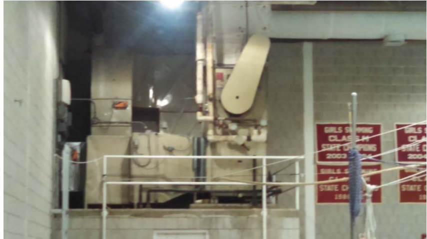
Pool Air-Handling Unit
