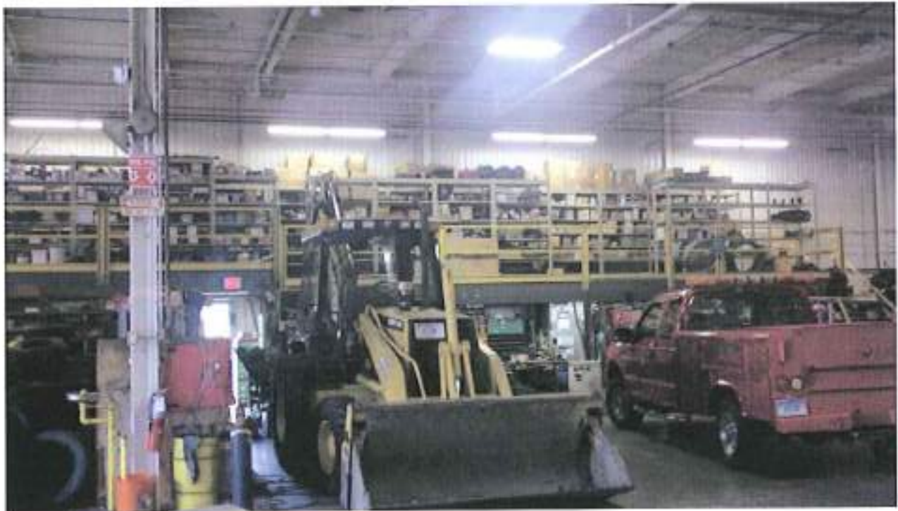
Vehicle Maintenance bays and parts storage are undersized to efficiently and safely support the operations
