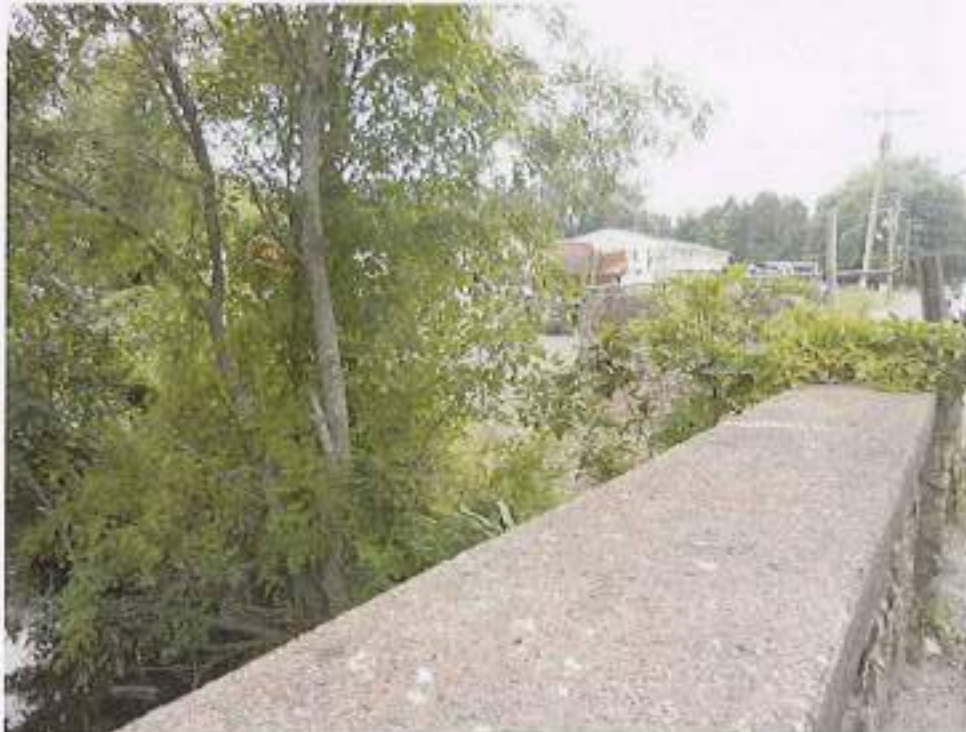
On bridge looking towards 114 School Ground Road site
