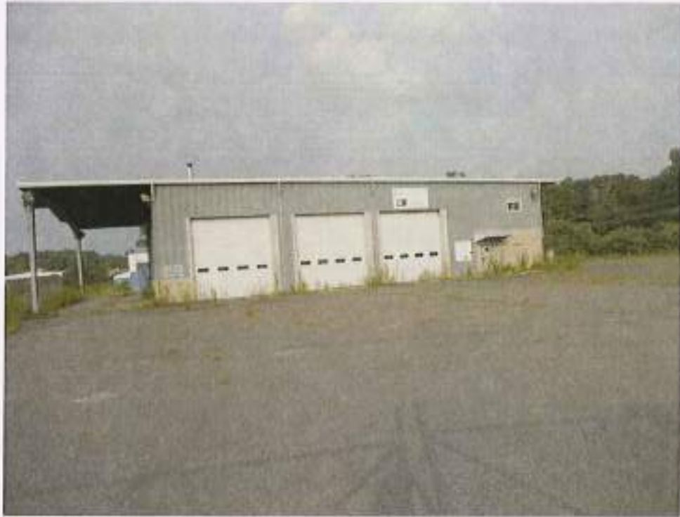
Buildings at 20 North East Industrial Road site
