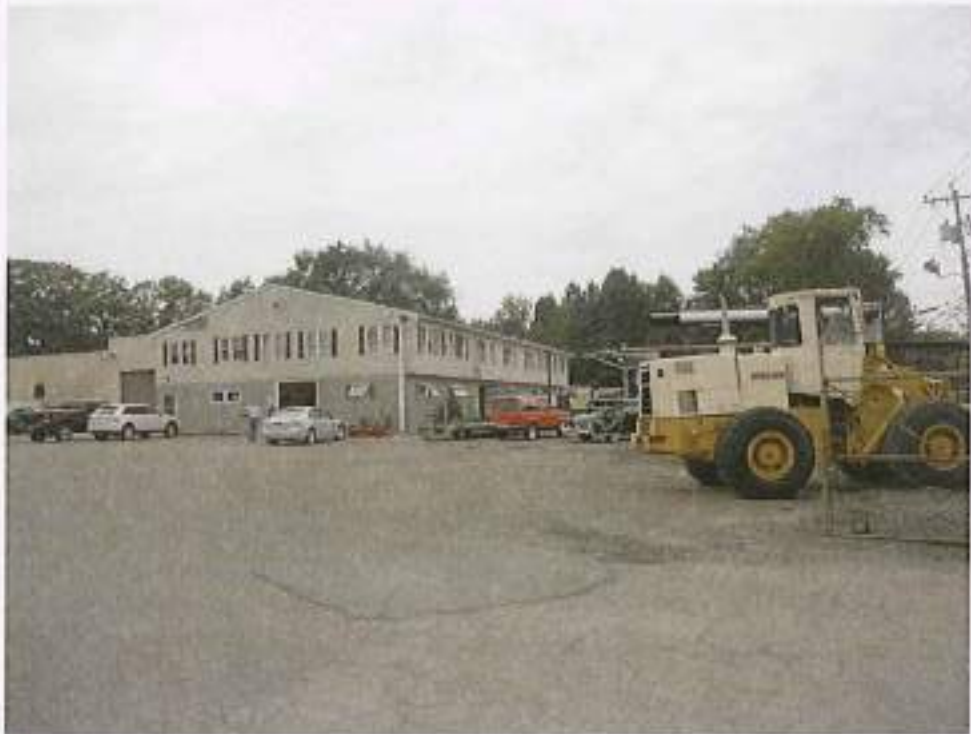
Building at 114 School Ground Road site
