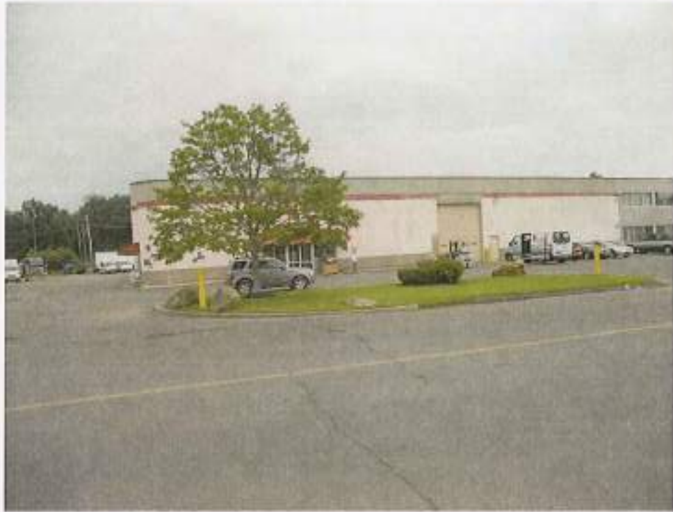
Front of building at 15 East Industrial Road
