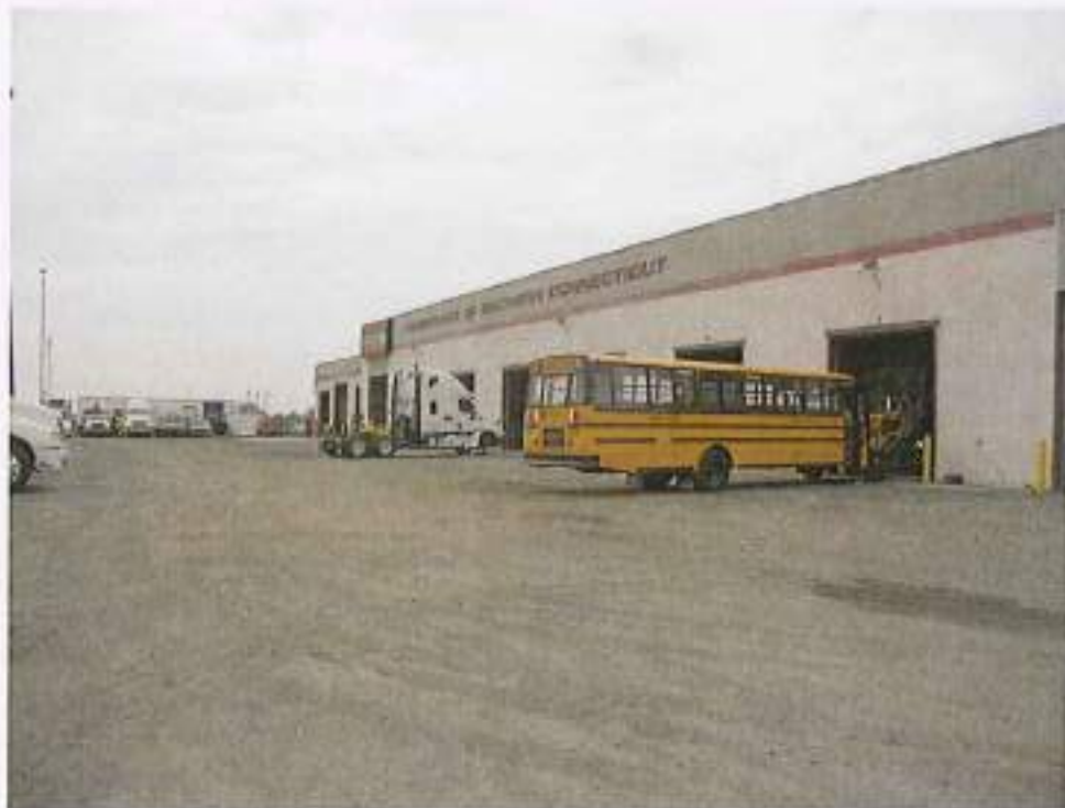
Back of building at 15 East Industrial Road
