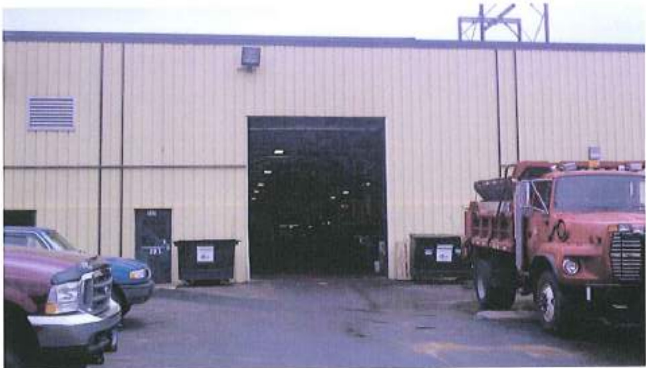
Inefficient single overhead door access to vehicle/equipment storage, workshops, material storage, and vehicle maintenance operations
