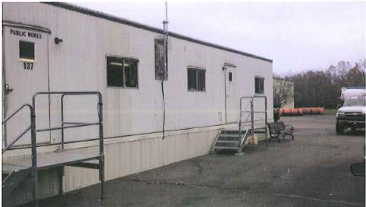
Rented facility is undersized resulting in staff operating out of temporary trailers
